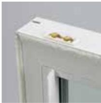
*Sash vent stops allow fresh airflow (lower right).*
