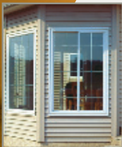
All Contractor series windows feature an integral J-channel for siding applications.
